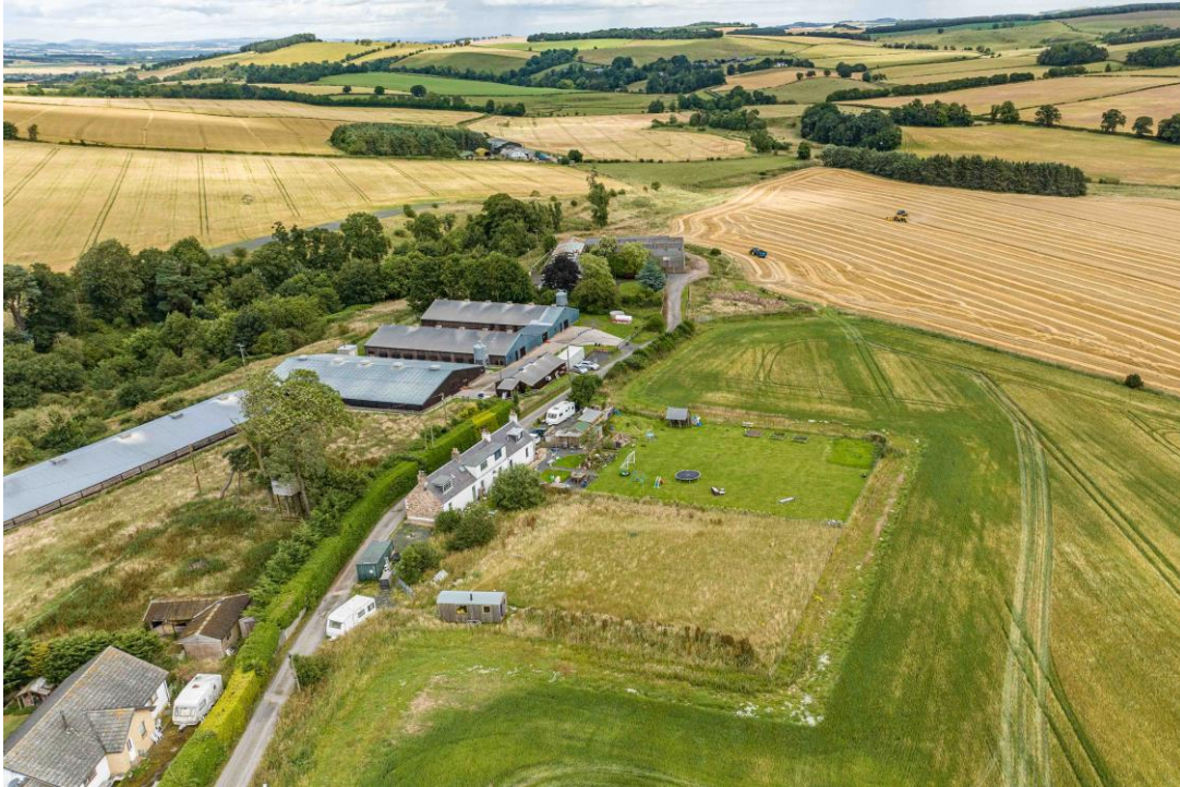
Figure 3: Aerial Photography of Existing Building Group
